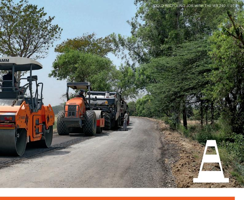
operation and accurate levelling guarantee optimum results. The machines in the WR series are ideally suited to applications in all performance ranges, from recycling thin asphalt layers on quiet minor roads to recycling up to 250mm-thick asphalt layers on heavily travelled motorways.
