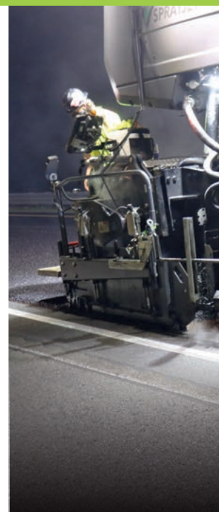
With the extra tank, a total of 1,875 gallons of bitumen emulsion are available for spraying.
