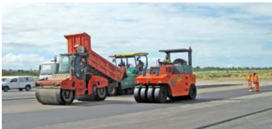
Vögele 1603-2 and three Hamm compactors on the Swaziland airport runway
