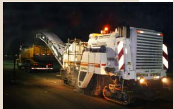
W 1900 carries out fine milling at Porto Alegre airport
