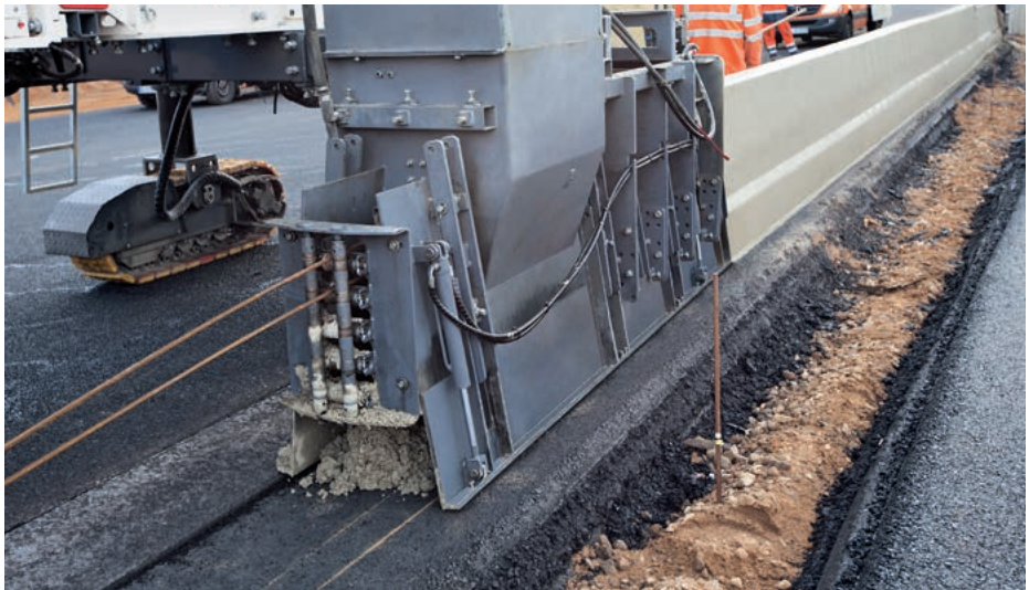
Paving a concrete safety barrier on an asphalt base
