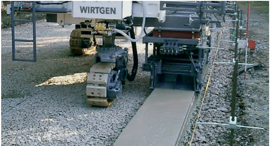
Paving a concrete profile on a base of crushed stone
