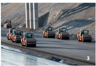
Hammtronic also contributes to the high productivity. The machine management system from HAMM optimizes both fuel consumption and the advance and vibratory drives of the rollers. The savings made are particularly evident in the operating costs when compacting large surfaces. This was the case on the motorway job site near Istanbul; the tandem rollers and the pneumatic-tyre rollers used for the project were equipped with Hammtronic.
