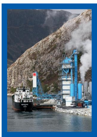
On site at the fjord: BENNINGHOVEN TBA mixing plant with cargo loading facility
