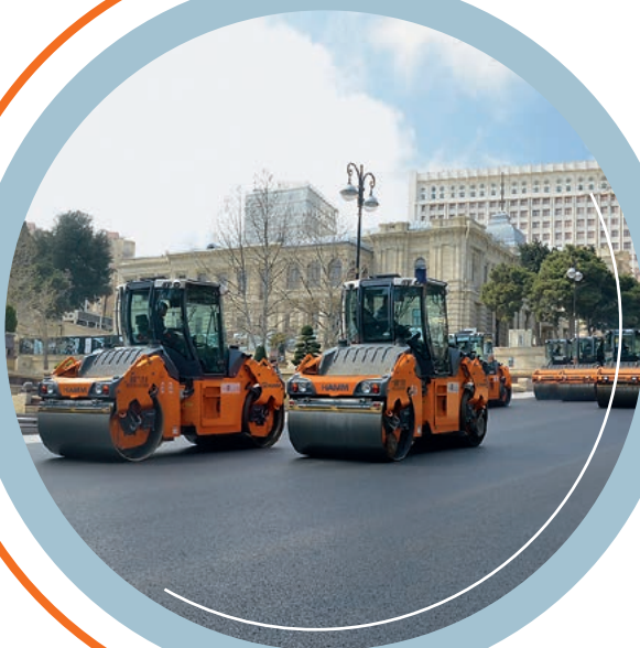
Constructing the Formula 1 track in Baku, Azerbaijan: when building this city circuit, a premium-quality asphalt surface had to be produced despite confined conditions as well as underground parking decks and pipelines. Oscillation rollers were therefore mandatory on this job.
