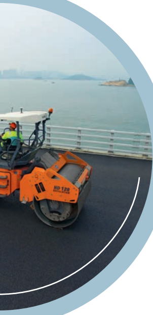
Construction of the Hong Kong-Zhuhai-Macao bridge in southern China: oscillation rollers dynamically compacted the thin asphalt overlay on the 35km-long bridge. The resultant surface was of outstanding quality, thanks to HAMM technology.
