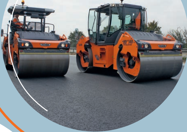
Construction of motorway section on the A61, Germany: oscillation rollers from HAMM achieved a high compacting performance and premium quality results.
