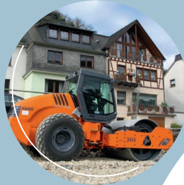
Earthworks between railway tracks and historic buildings in Oberwesel, Germany: just one oscillation roller could deliver the required compaction here without damaging the half-timbered houses or the sensitive railway tracks.
