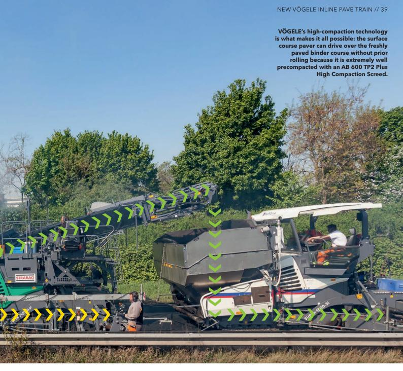
Road rehabilitation at top speed: the new "Dash 3" generation of the InLine Pave train shows just what it can do in practice. The unique combination of cutting-edge VÖGELE technologies lays the binder and surface courses in a single pass - a method which makes this recognized construction method particularly economical, too.
