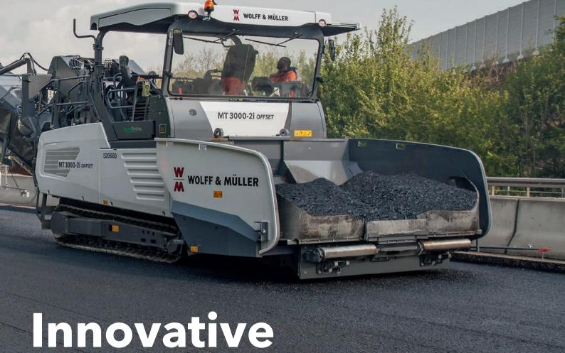
First job for two MT 3000-2i Offset PowerFeeders fresh out of the factory: the VÖGELE PowerFeeders supported the 3 SUPER pavers rehabilitating the carriageways at the Weinsberg motorway intersection. The advanced machines ensured a consistently high flow of mix for a continuous paving process.
