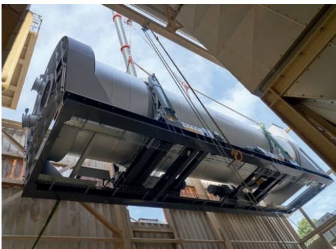
Retrofitting a REVOC system
