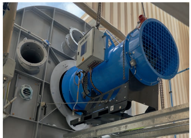
Retrofitting a MULTI JET multi-fuel burner
