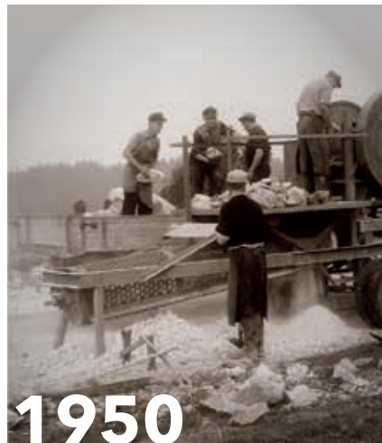
Hand-fed wheeled mobile jaw crusher with drum screen from KLEEMANN.
