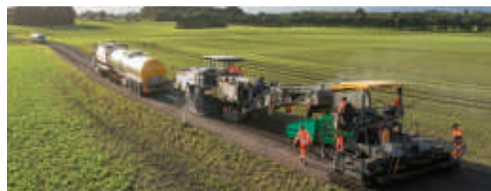
The W 380 CR (i) from the CR series during the cold in-place recycling of a road surface in a single pass.
