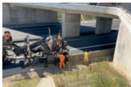
Paving of a concrete safety barrier including reinforcement with the slipform paver SP 33.
