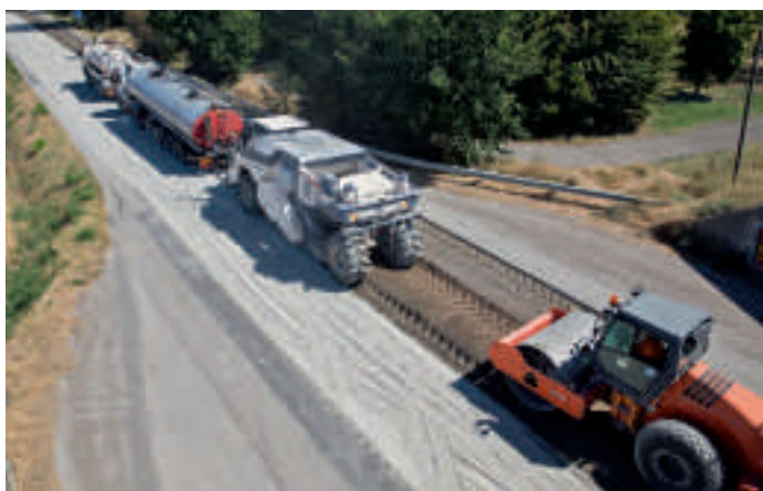
Production of a new, high quality base layer with the WR 240 (i) from the WR series.
