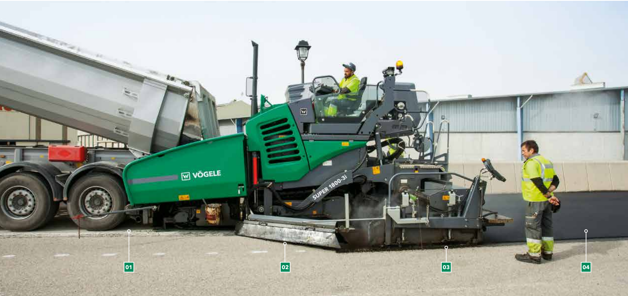
Hot bitumen emulsion at a temperature between 158 to 176 °F (70 to 80 °C) is applied by the spray paver.
