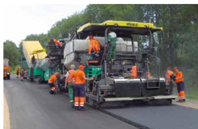
Pavement rehabilitation of a national road, pave width 3.75 – 5.25 m: Rehabilitation in single-lane width. Traffic kept flowing on the adjacent lane. Slope of 2%. Referencing from the milled base using the Big MultiPlex Ski allows for paving to the highest standards of evenness.
