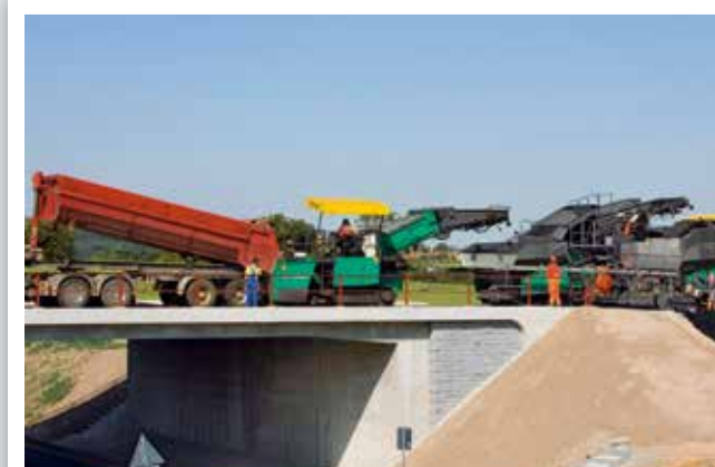
New construction of a federal highway, pave width 7.5 m: Two-layer paving between 6 bridges. On the bridge decks asphalt was placed by the paver for surface course. VÖGELE Big MultiPlex Ski used for grade and slope control.
