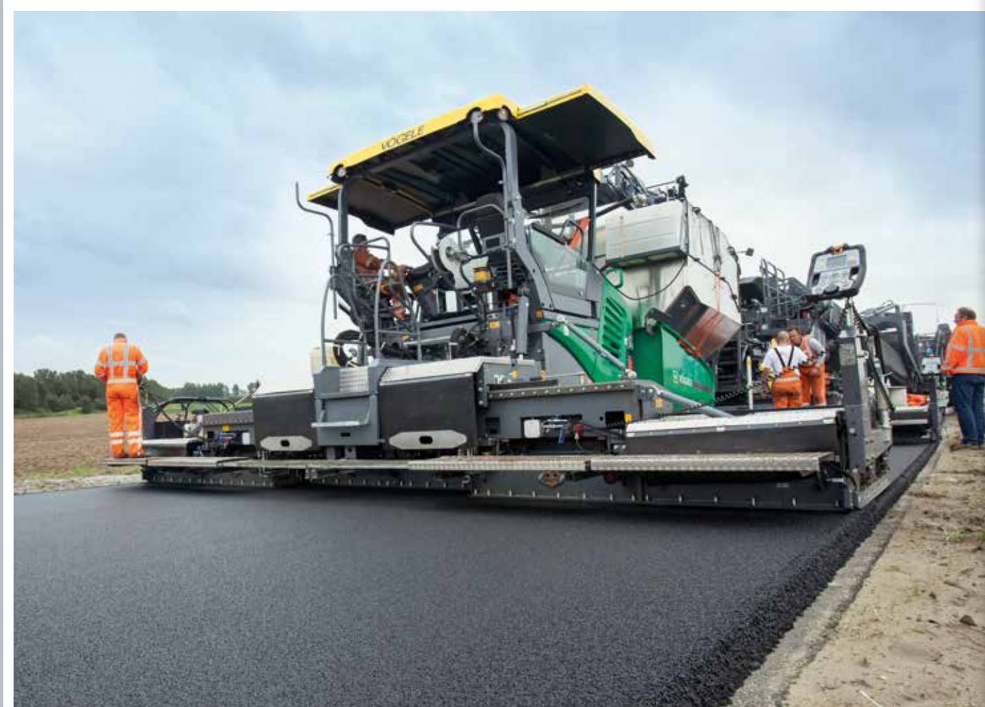
Due to the two pavers' auto-levelling properties, InLine Pave achieves evenness at the highest level.
