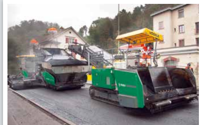
Pavement rehabilitation of a rural road, pave width 5.5 – 7 m: 9.5 cm binder course and 2.5 m surface course were paved in 12-hour shifts – no problem for the InLine Pave train.
