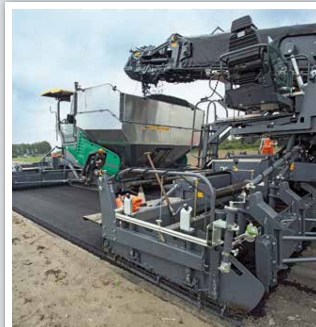
By way of the transfer module on the paver placing binder, surface course mix is conveyed to the second paver following behind.
