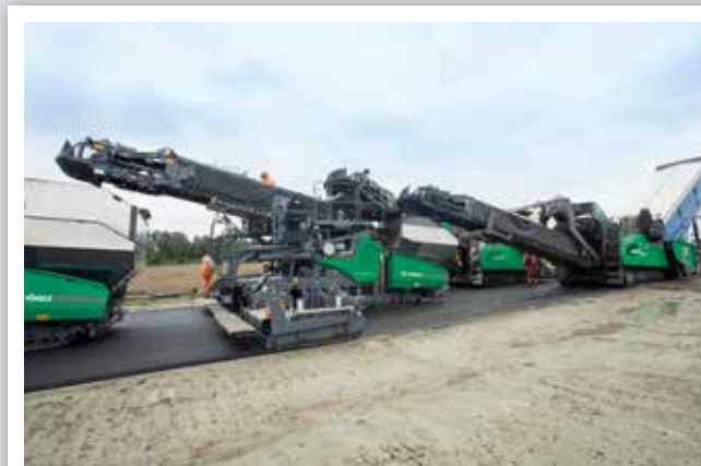
Pavement rehabilitation of a federal highway, pave width 7.5 m: Thanks to its large pave width and high pave speed the InLine Pave train was supplied with material from two PowerFeeders simultaneously.
