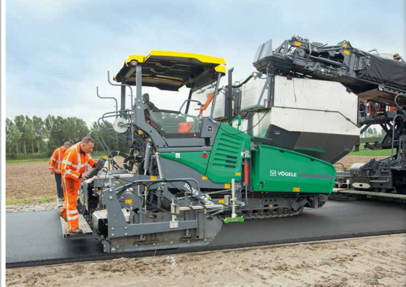
An extra material hopper holding 25 tonnes stores a large quantity of surface course mix.
