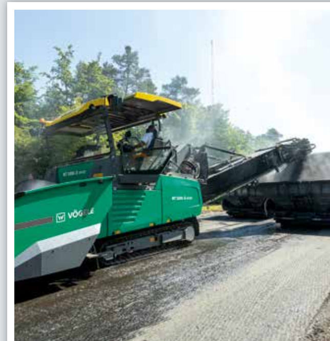
The feeder operator has an unimpeded view of the feed vehicles and the SUPER 2100-3i IP.
