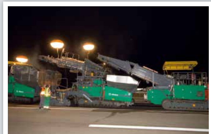
Pavement rehabilitation of a motorway, pave width 4.7 m: The roadworks on the busy motorway were carried out at night.
