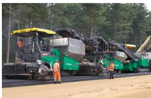
New construction of a motorway, pave width 5m: Before placing binder and surface courses, the base course had been built with the SUPER 2100-2 IP.
