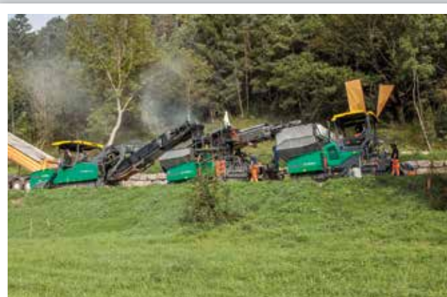
Pavement rehabilitation of a federal highway, pave width 7 m: Seamless pavement rehabilitation of a federal highway with curve radii of less than 200 m.
