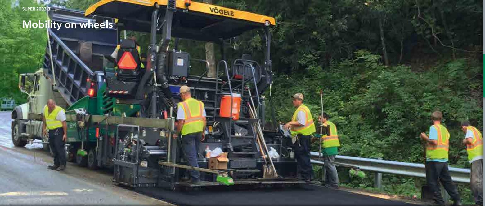
One of the SUPER paver's strong points is its excellent traction behavior. Separate drive and electronic control provided for each powered wheel ensure constant straight-line travel and accurate turns.
