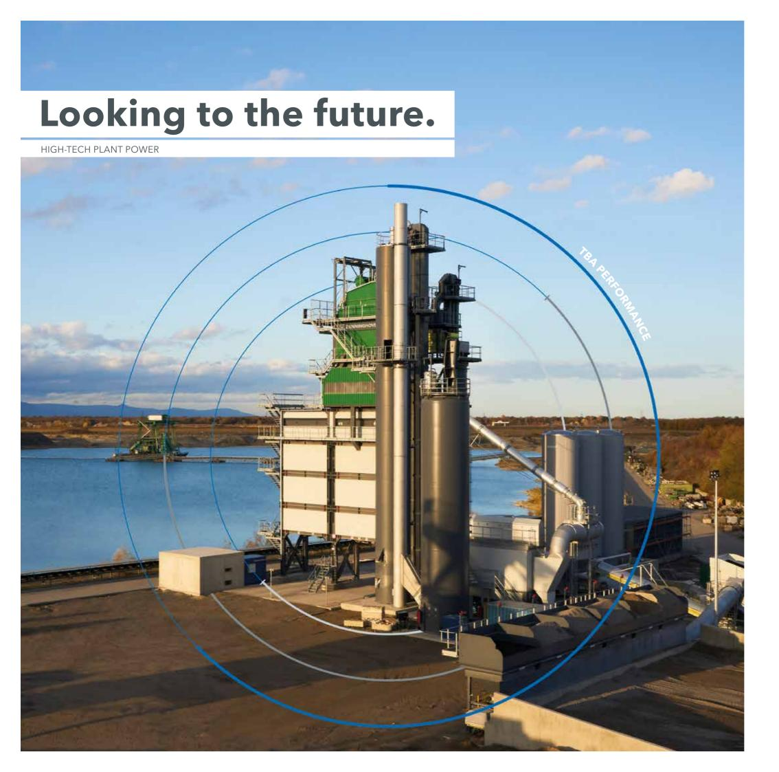
The compact TBA plants feature strong and reliable plant performance during operation. Optimum quality of the asphaltic mixture is always guaranteed with a mixing capacity of up to 320 t/h.
