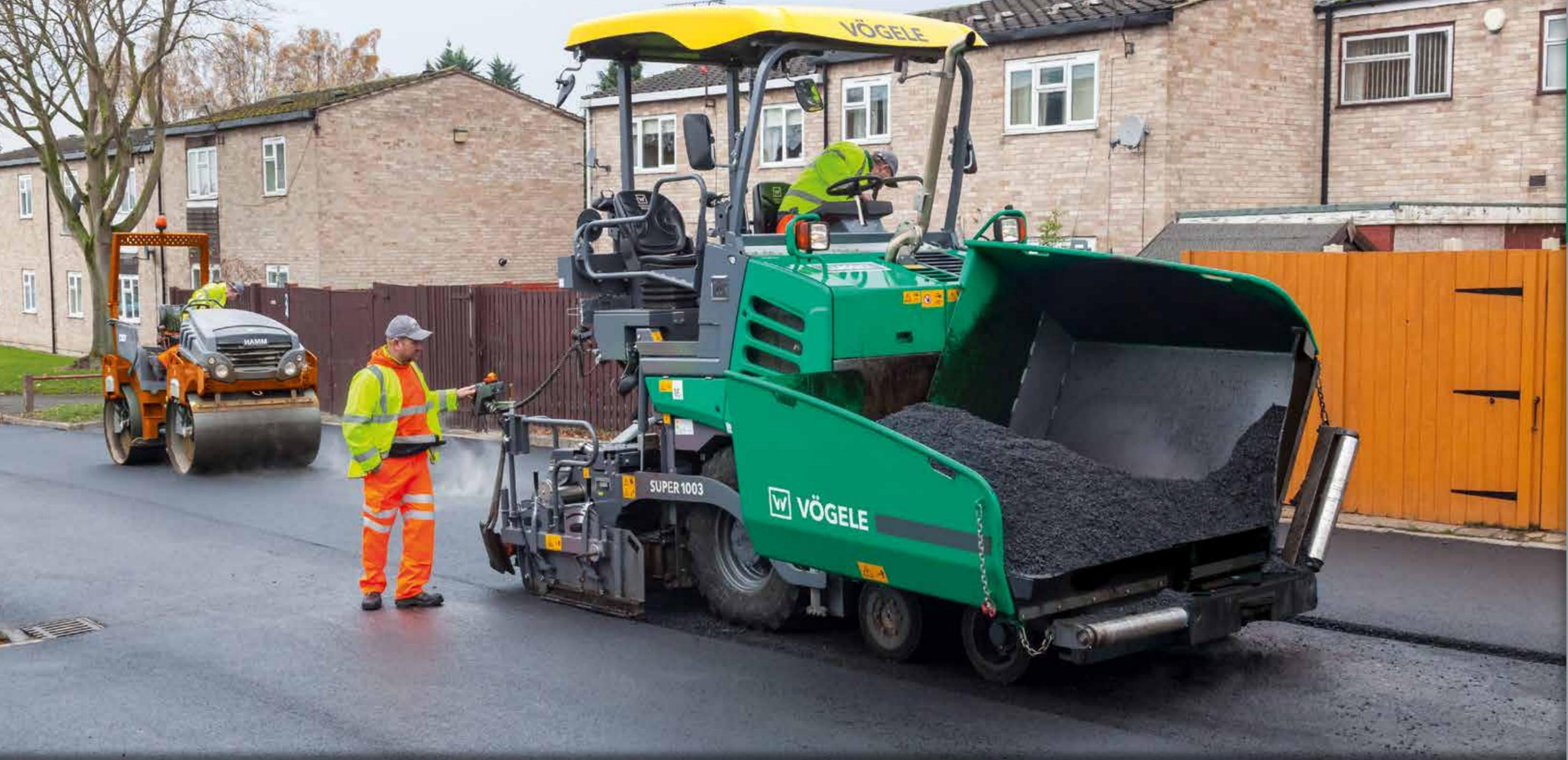
**A continuous flow of mix** is key to ensuring uninterrupted and high-quality paving. That is why we attach such importance to professional material management when designing our pavers.
