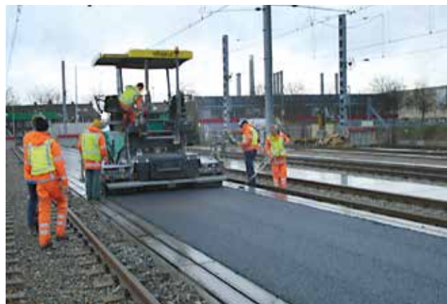
ASPHALT PAVING ON RAILWAY PLATFORMS
