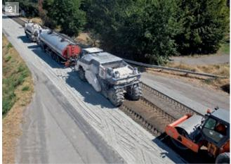
Their tremendous engine power enables the WR 240i machines to push the two tanker trucks travelling ahead which deliver water and bitumen emulsion to the recycler via coupled hose connections.
