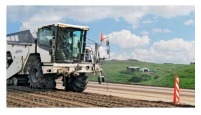
The WR 250 pulverizes the existing pavement material and added gravel at a working depth of up to 56 cm.
