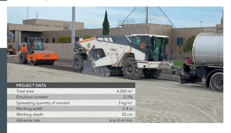
The WR 250 injects emulsion and water into the mixing chamber via injection bars installed in the front part of the rotor housing.
