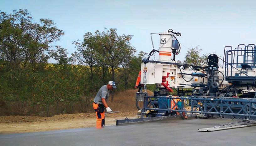
The inset slipform paver is the perfect choice for the cost-effective paving of large concrete surfaces ranging from 16 ft to 40 ft wide and 18 in (450 mm) thick.
