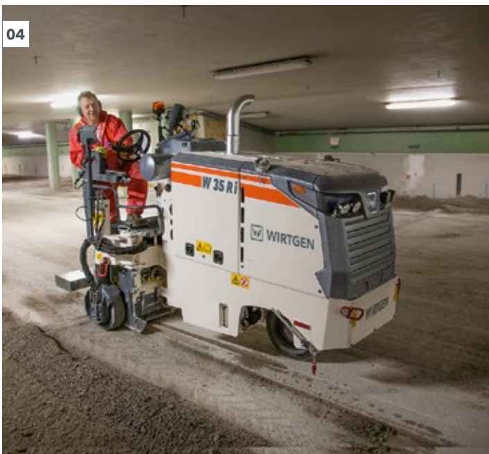
01 Milling a sidewalk.
