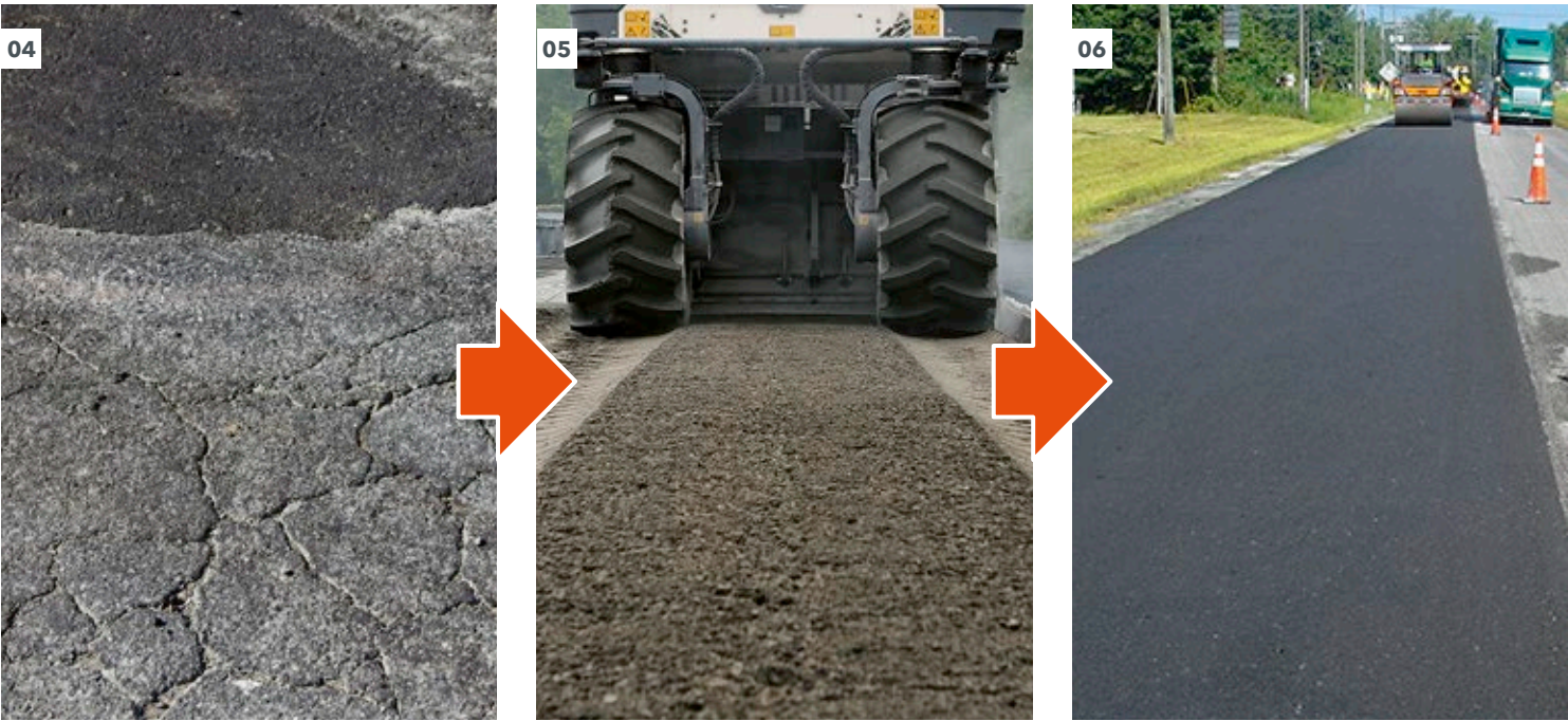
04 – 06 In cold recycling, damaged asphalt layers are granulated, mixed with binding agents, compacted, and repaved.
