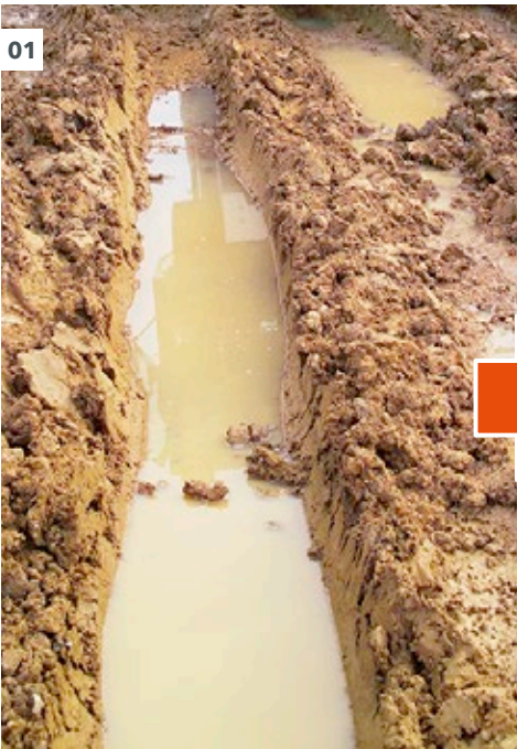
01 - 03 Stabilization transforms sub-bases with insufficient bearing capacity into soil that is suitable for paving and compaction.
