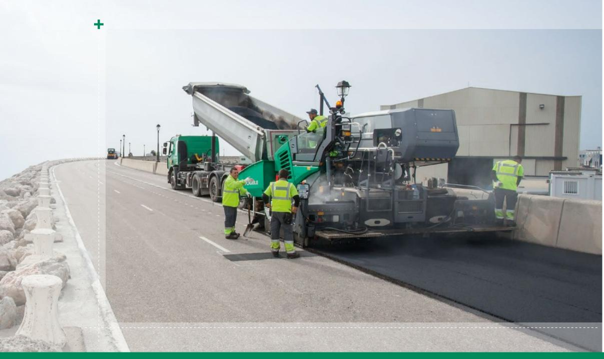
Paving thin layers using unique spray technology **Conventional paving** of binder and surface courses
