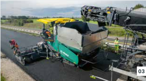
By way of the transfer module on the paver placing binder, surface course mix is conveyed to the second paver following behind.
