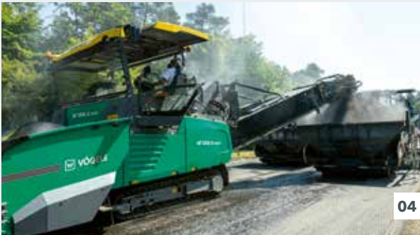
The feeder operator has an unimpeded view of the feed vehicles and the SUPER 2100-3i IP.
