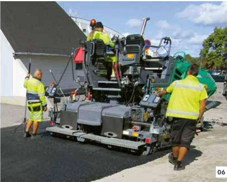
04 The paver operator's platform ensures maximum visibility. 05 Optimum feeding with mix thanks to the large material hopper. 06 Can be combined with the AB 340 Extending Screed.
