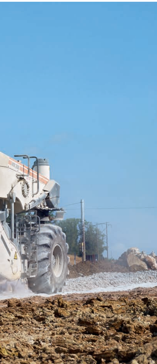
5 | During soil stabilization operations, either cement or lime is pre-spread as a binding agent.
