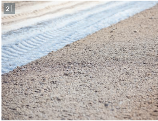
2 | Soil mixed with a binding agent can be easily compacted.
