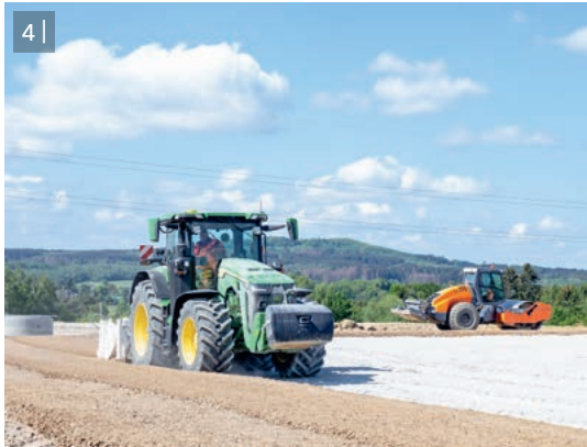
5 | During soil stabilization operations, either cement or lime is pre-spread as a binding agent.
