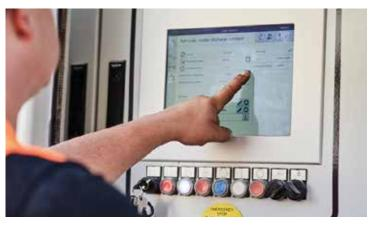
> Trigger the "Lock rotor" command via SPECTIVE
