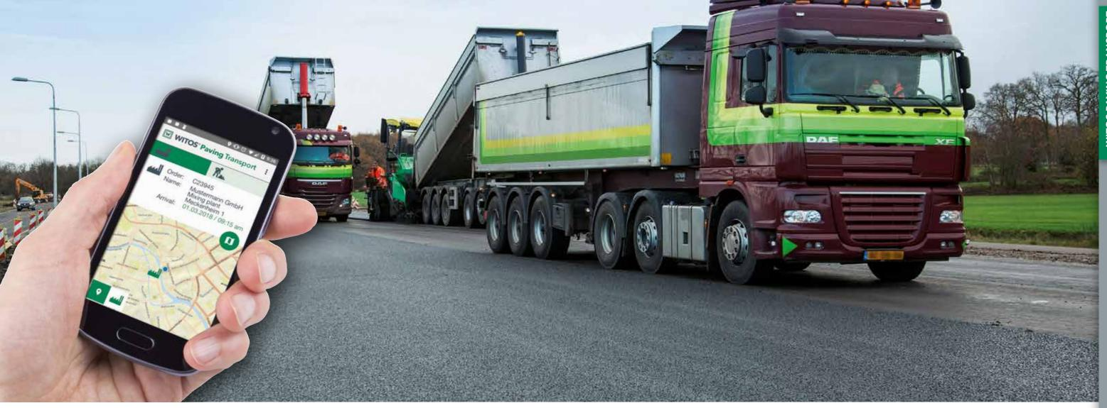
Thanks to WITOS Paving Plus the paving team, site manager and mixing plant receive real-time information on the arrival of mix lorries at the job site throughout the construction period.
