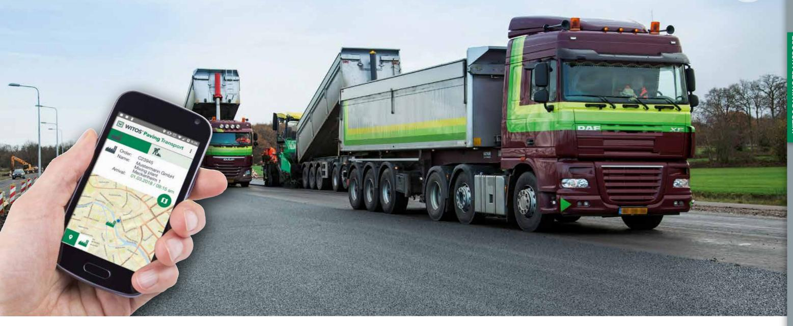
Thanks to WITOS Paving Plus the paving team, site manager and mixing plant receive real-time information on the arrival of mix lorries at the job site throughout the construction period.
