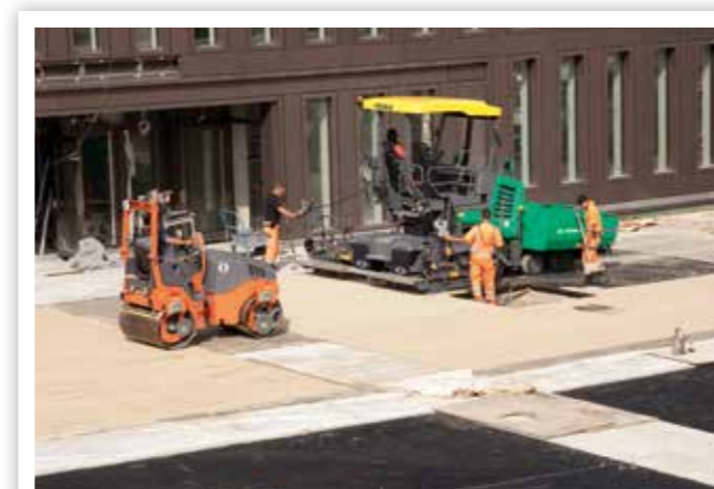
ASPHALT PAVING ON COMMERCIAL SITES
