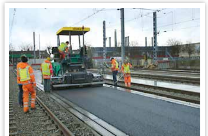
ASPHALT PAVING ON RAILWAY PLATFORMS
