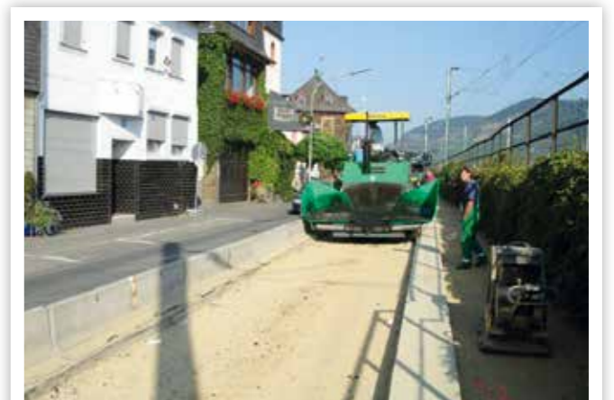
PAVEMENT REHABILITATION ON MUNICIPAL ROADS
