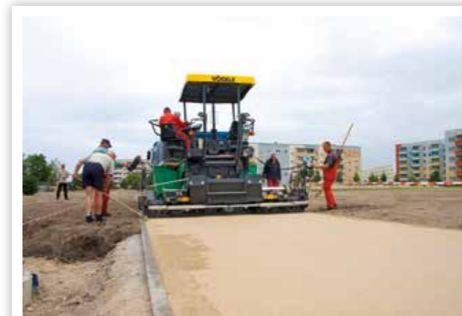
PAVEMENT REHABILITATION ON ACCESS ROADS
